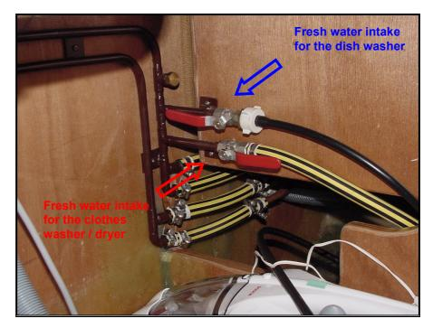
Picture 101 – Fresh water intakes stop cocks for the clothes washer / dryer and dish washer (photographed open)
