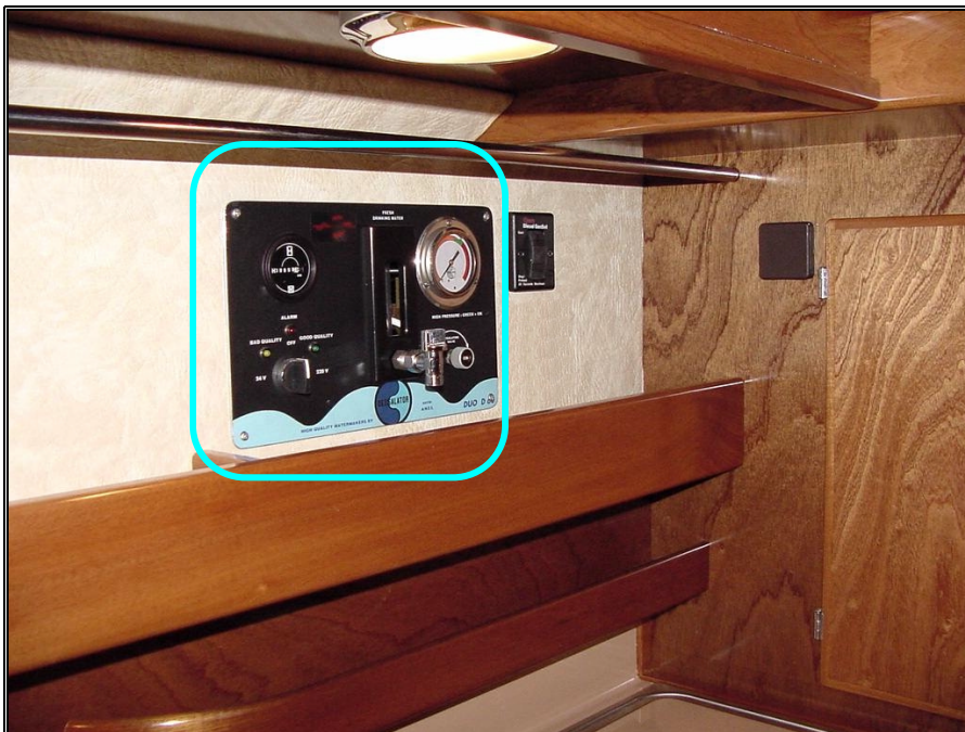
Picture 6 – Desalinator control panel
