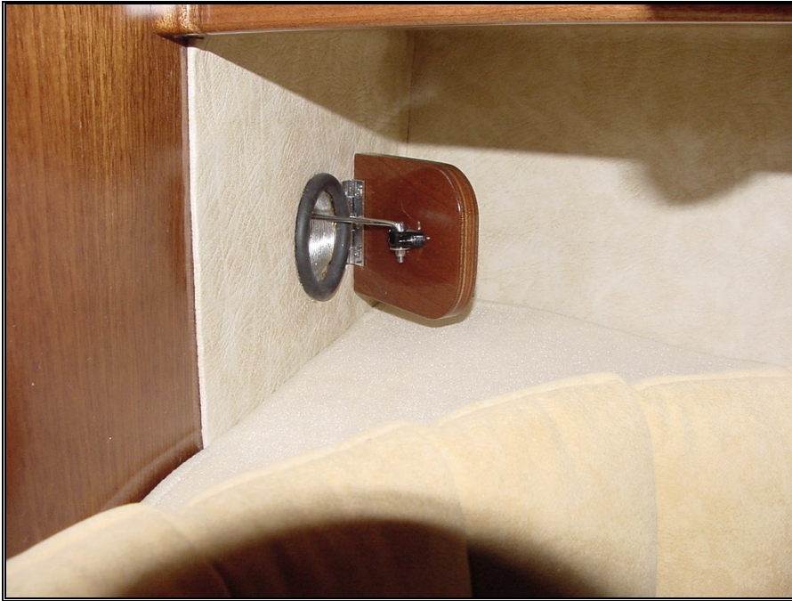
Picture 24 – Fresh air outlet in the fore cabin
