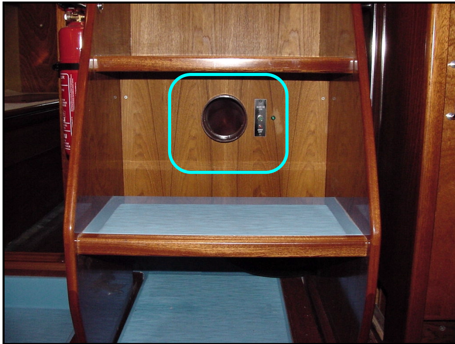
Picture 22 – Fresh air outlet in the saloon and circuit breaker
