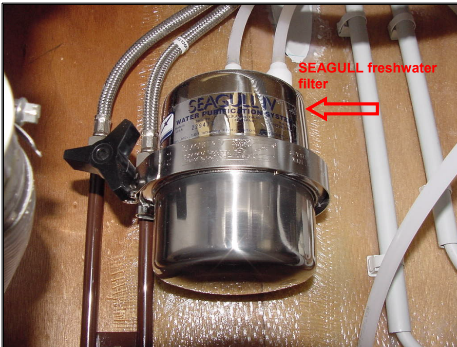
Picture 31 – SEAGULL IV freshwater filter
