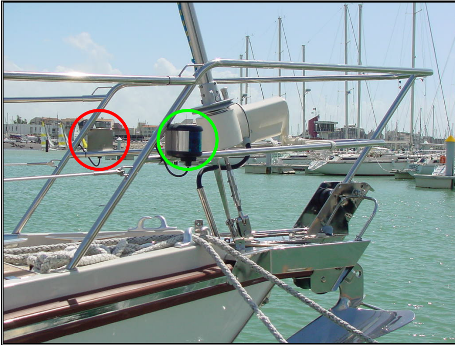
Picture 27– Fore DHI deck navigation lights
